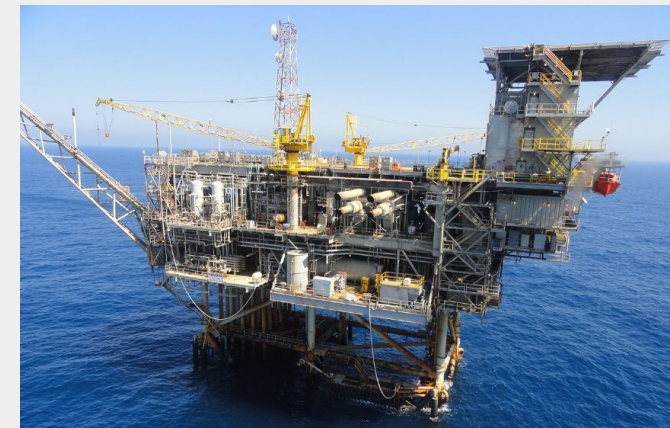
Green Canyon 18A Production Facility
