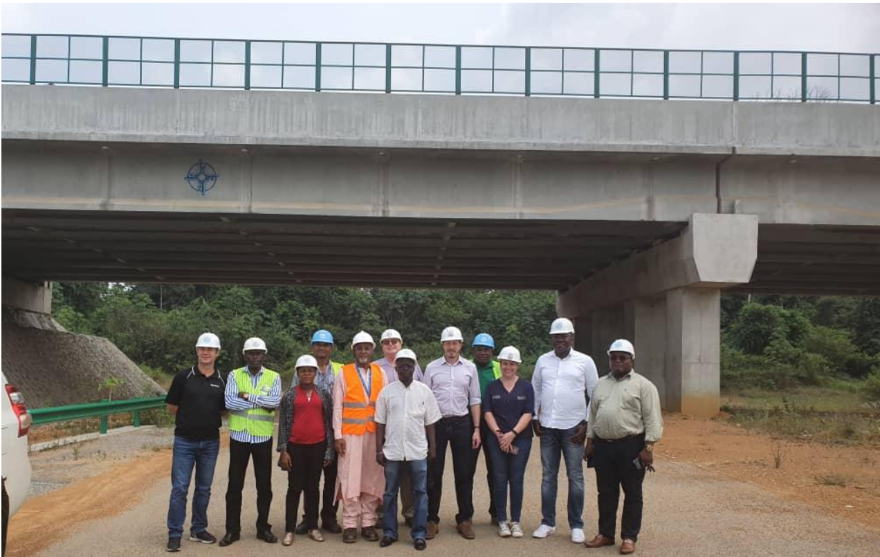
Figure 5 – Canyon’s study and development team reviewing the transport corridor allocated for the future rail link to the Kribi Port.
