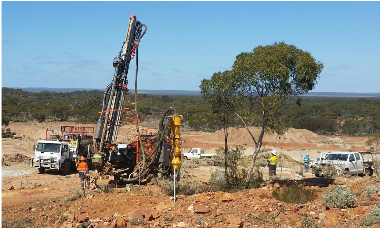
Figure 2: Commencement of grade control drilling at Boorara
