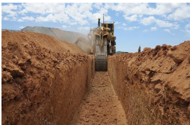
Initial cut of the box-cut top bench
