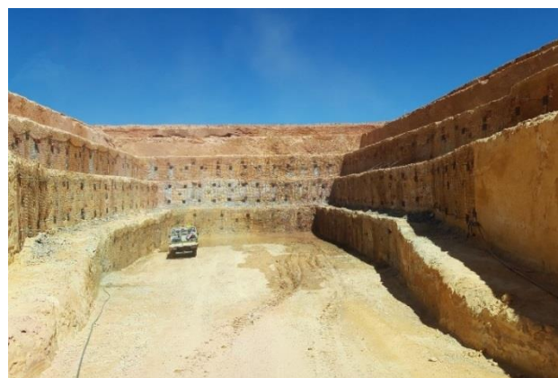
Completed headframe box-cut
