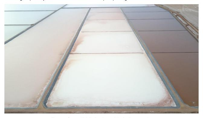
Figure 6: Stage 2 Kainite Ponds precipitating harvest salts
