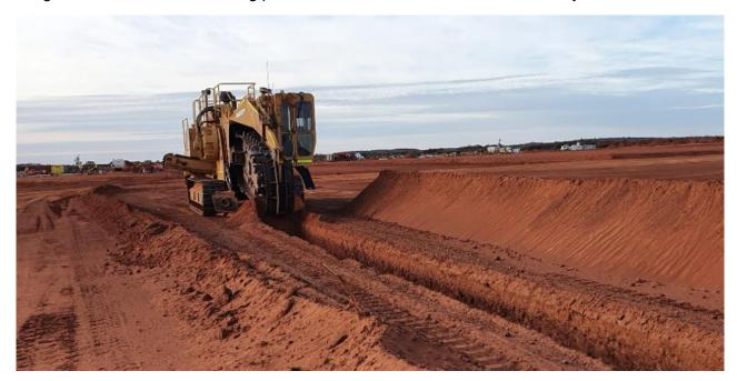
Figure 11: Excavation of trenches with a Vermeer at the Process Plant & Village site
