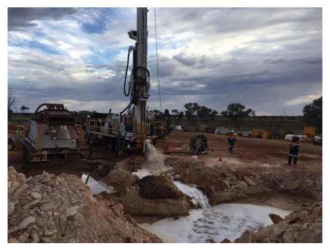
Figure 18: Airlifting of Monitoring Bore at Pad 17
