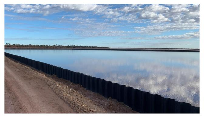
Figure 3: Stage 2 Ponds lined with PVC sheet piles
