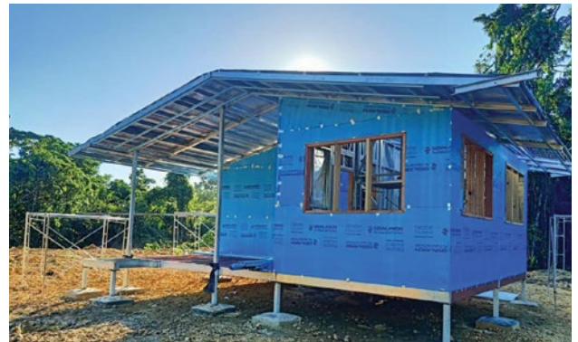
Figure 11: New house under construction
