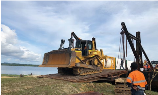
Figure 5: Equipment for Civil Works Program barged to site
