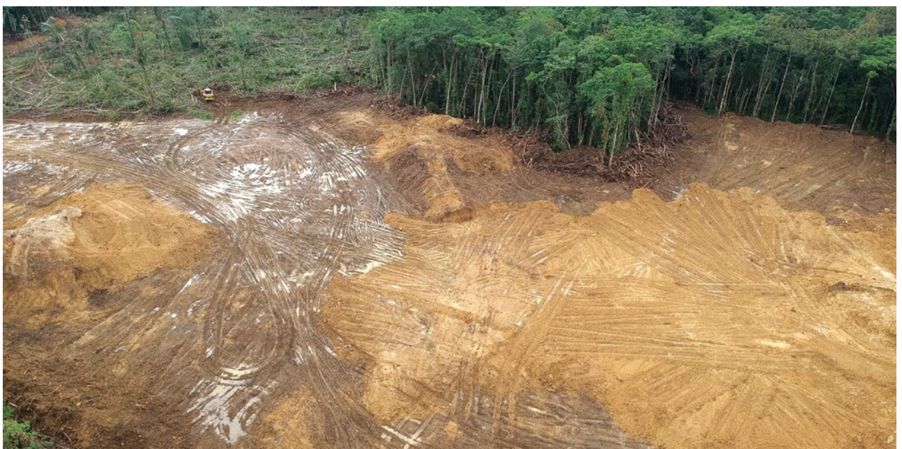
Figure 7: Process plant site cleared as part of the Civil Works Program
