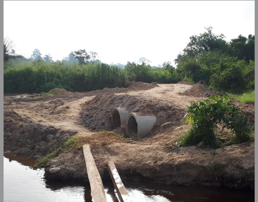
Low cost bridge works expected to be completed by 15 May 2020
