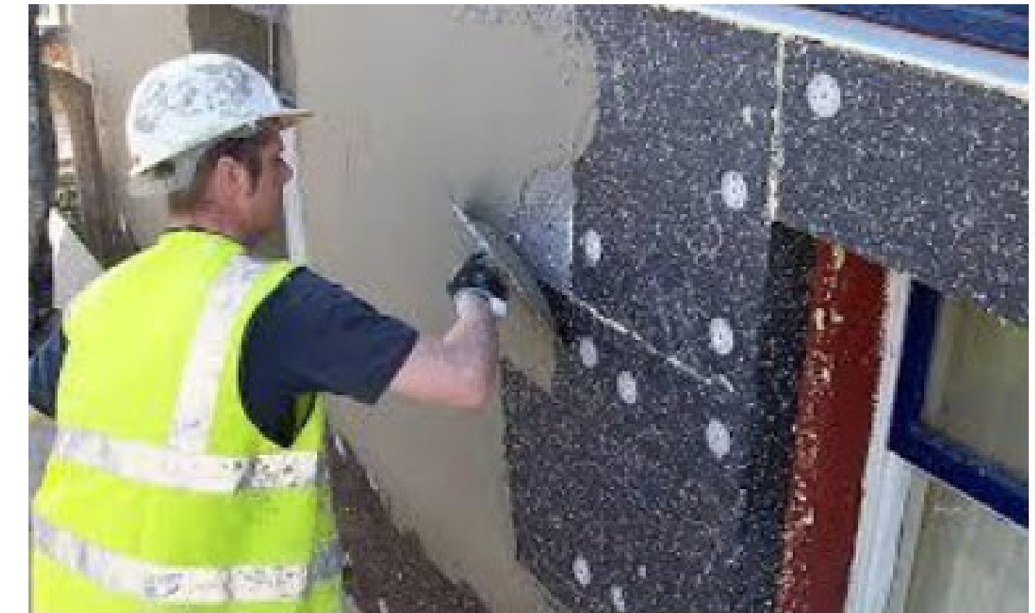
Installing Flame Retardant Foam
