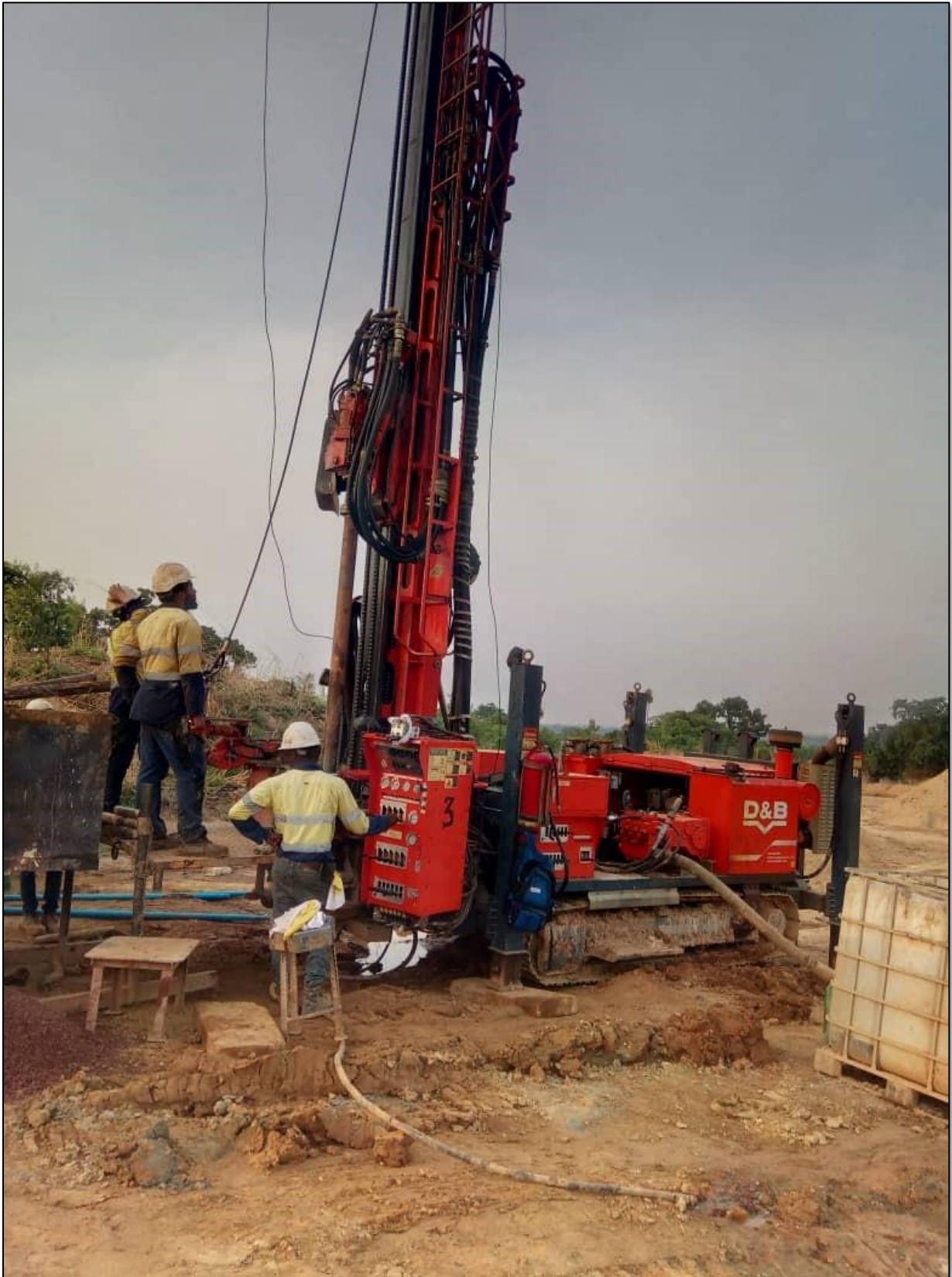
Figure 1 – Diamond drill rig to be used at Kaninko (drilling on a nearby mine site)
