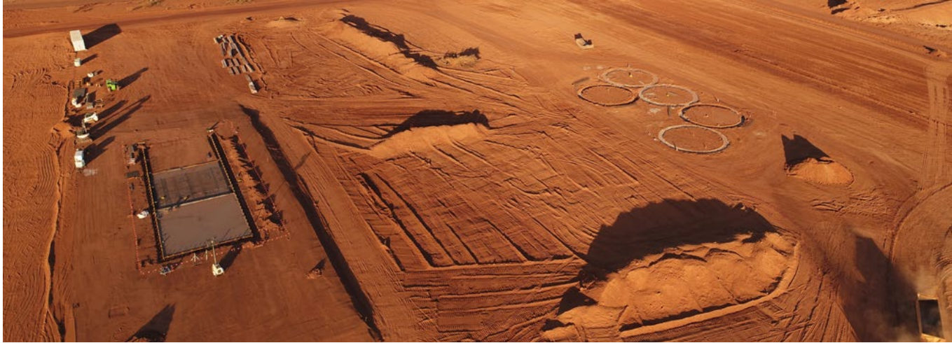
Civil earthworks for processing plant
