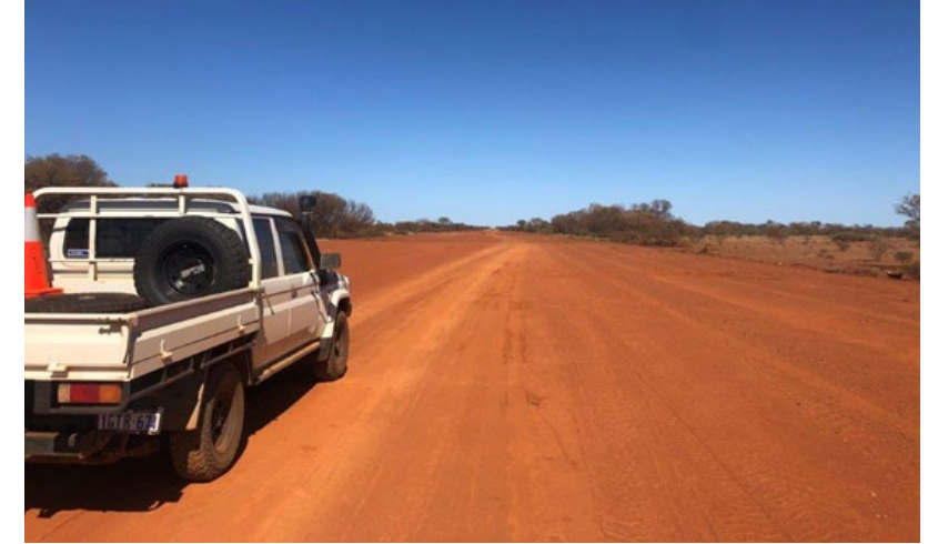
Access road construction
