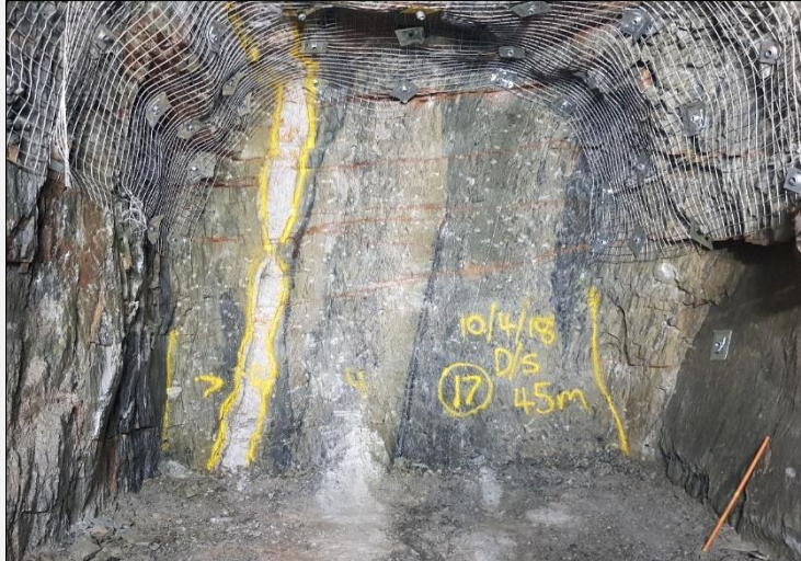
Second Fortune underground development drive, Level 2
