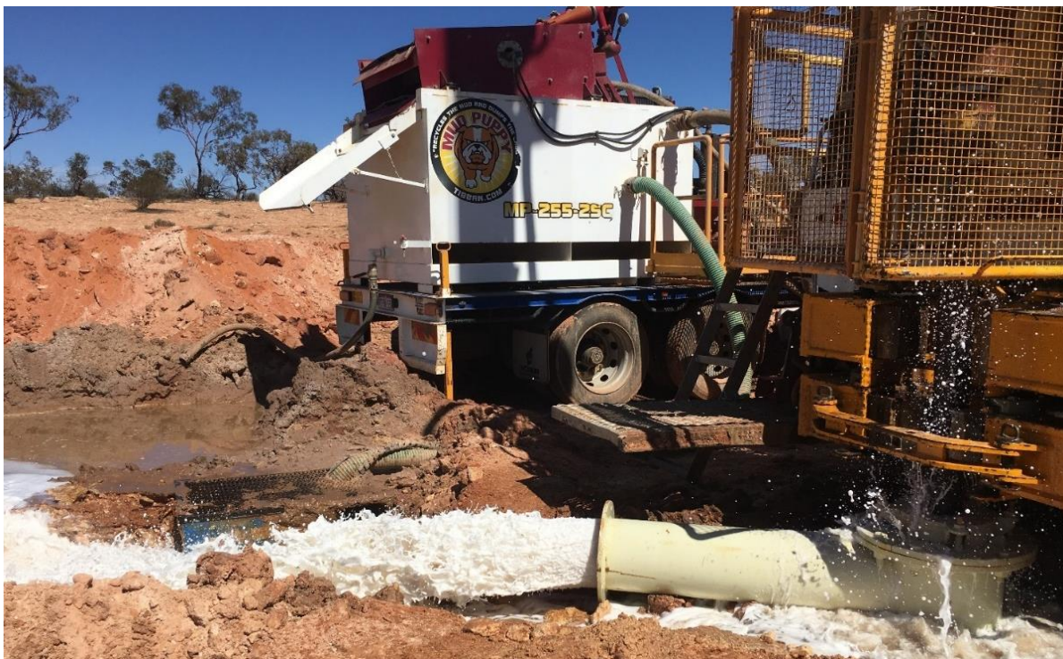
Figure 2: Airlift development at Pad 17
