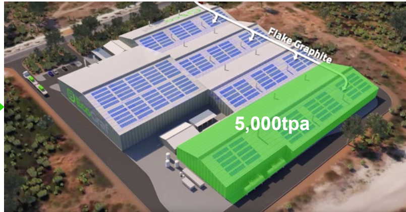
Staged expansion from 5,000tpa to 20,000tpa
