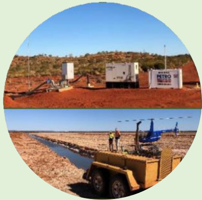
Bores and Trenches Brine Pumping
