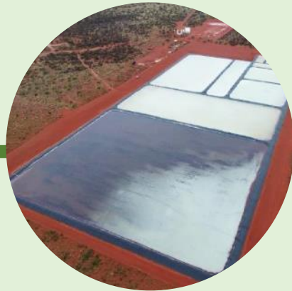
Brine Solar Evaporation
