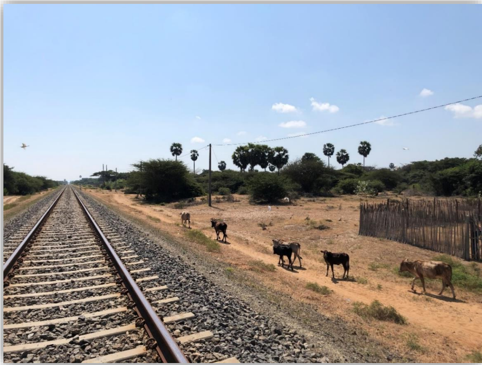
Figure 12 Rail track on Mannar Island that connects to the mainland network.
