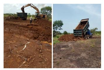
Initial mining and stockpiling of oolitic iron ore with Sunday Awoyemi (KCM geologist) on grade control duties. (Note: low strip ratio with iron ore at or near surface)
