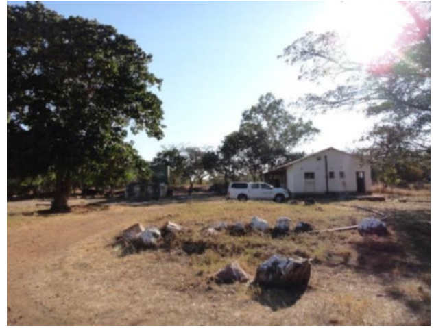
Dunrobin mine offices
