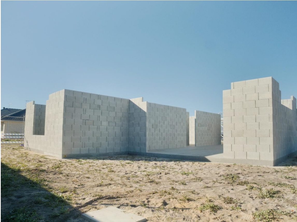
The completed structural walls at the Dayton site
