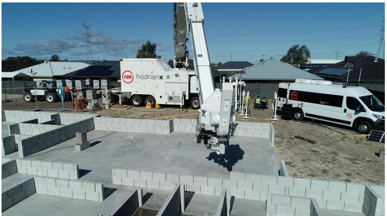
The Hadrian X@ building its first display home in Dayton, Western Australia
