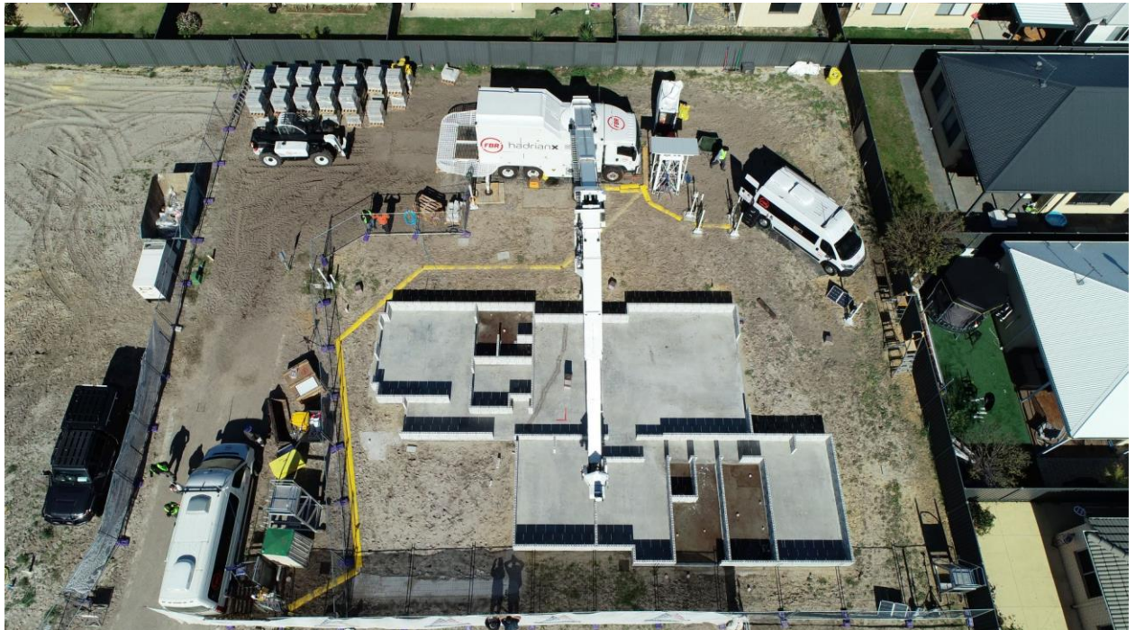
Aerial view of the Hadrian X@ building its first display home
