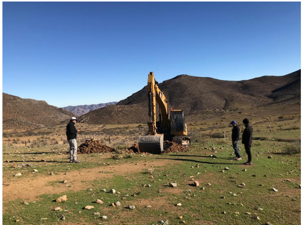
Figure 1: Excavator on site at Colina2 Gold Copper Project
