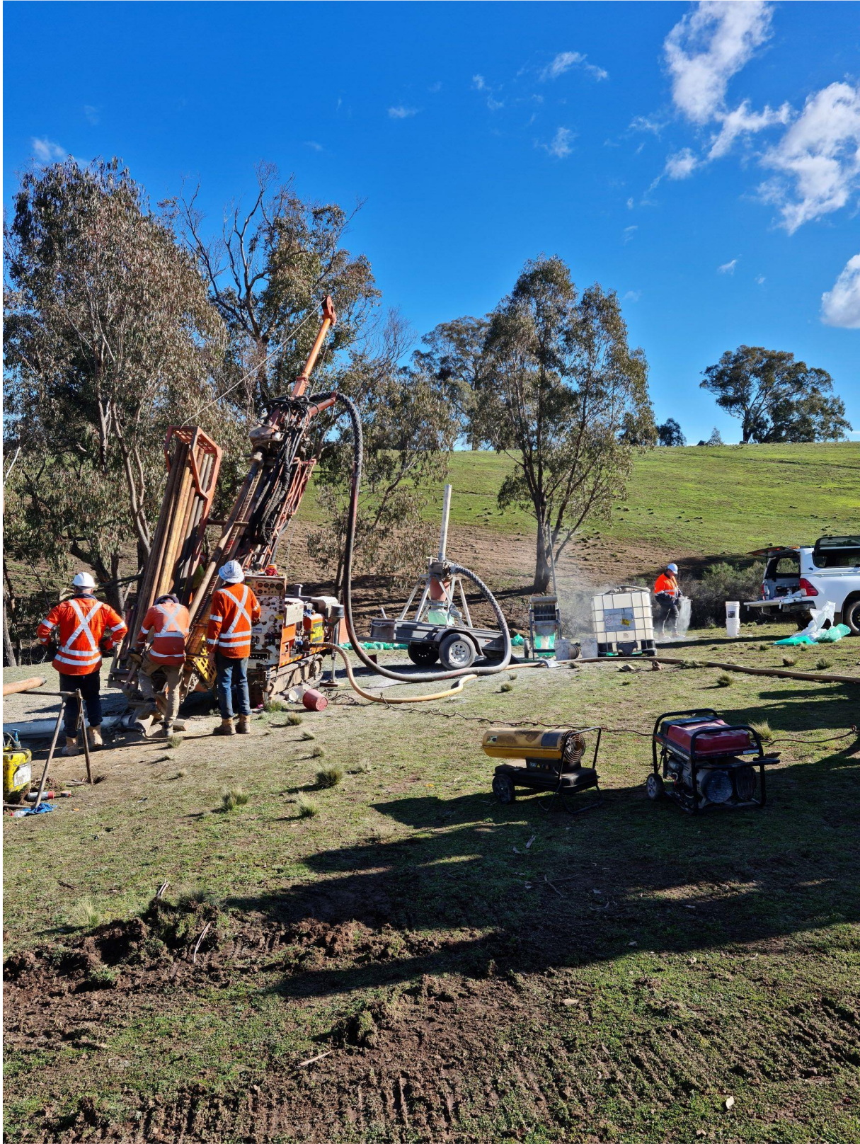
Photo 1 Drill Rig at Kempfield on drill hole AKRC205 on the contact of the Cu-Au footwall zone
