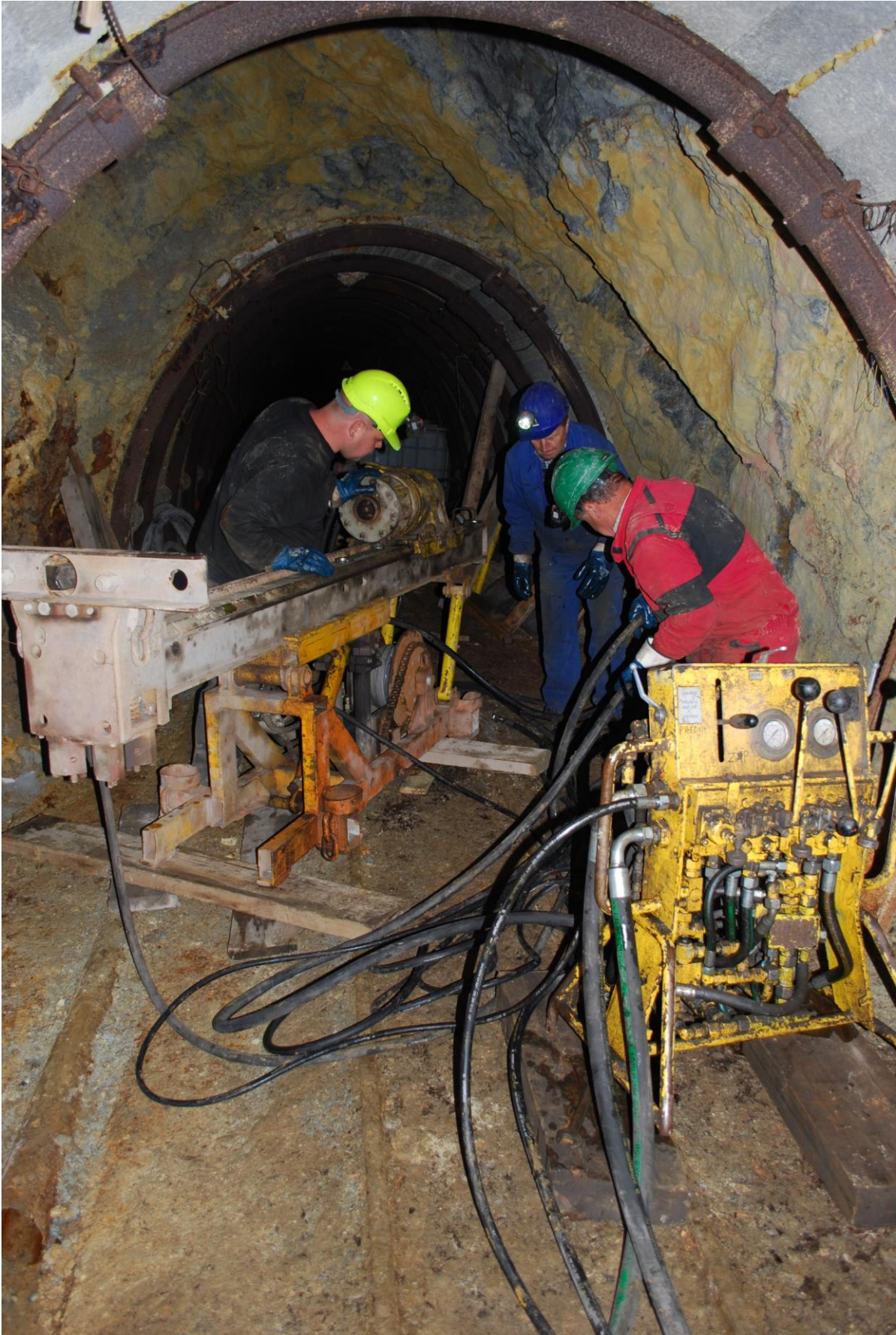
Image 4: Drill rig and ancillary equipment being set up at the drill site within the underground Andrej adit
