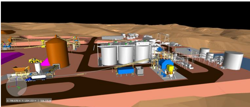
View to the south of the revised Borborema plant layout (2020), showing grinding circuit, CIL tanks and fine ore bin/emergency stockpile feeder to the left
