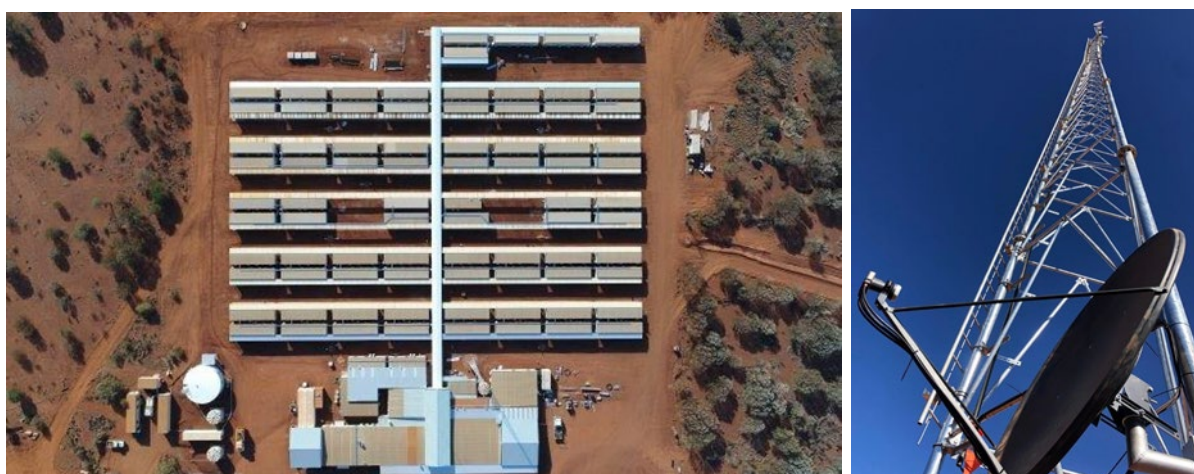
Installation of the accommodation village and communications tower
