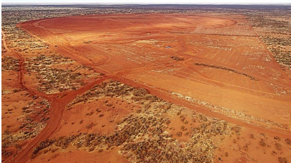
Clearing and topsoil removal for the TSF/IWL
