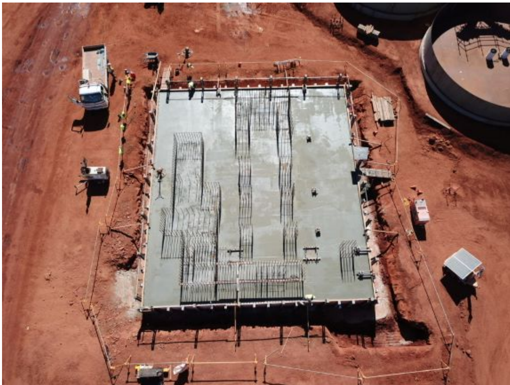
Ball mill foundations
