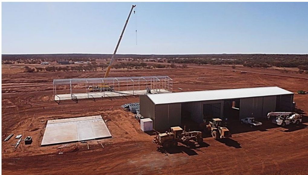
Maintenance workshop, maintenance office concrete foundation and stores shed erection
