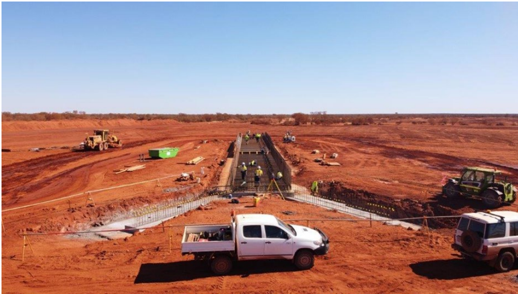
Fine ore stockpile tunnel concrete footing
