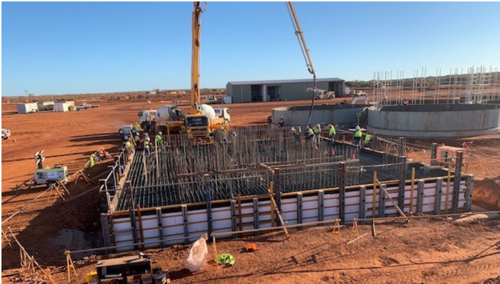
Pouring of concrete foundation for ball mill
