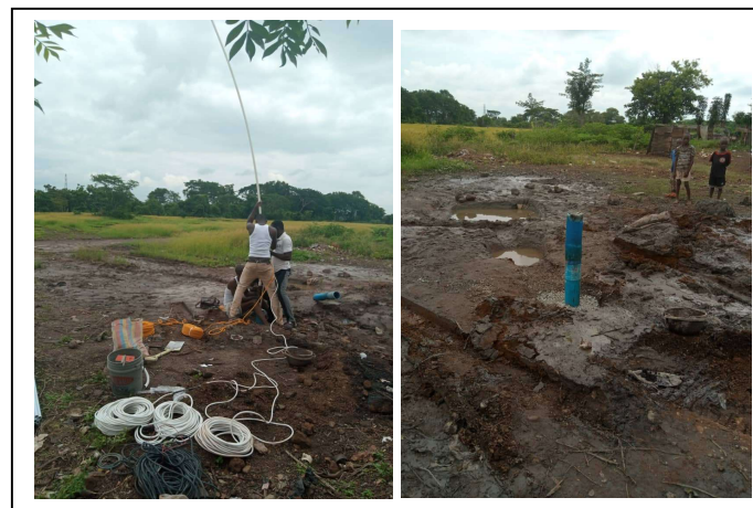
Casing the water well and lowering the pump (LHS). Newly drilled, cased and collared water well (RHS)
