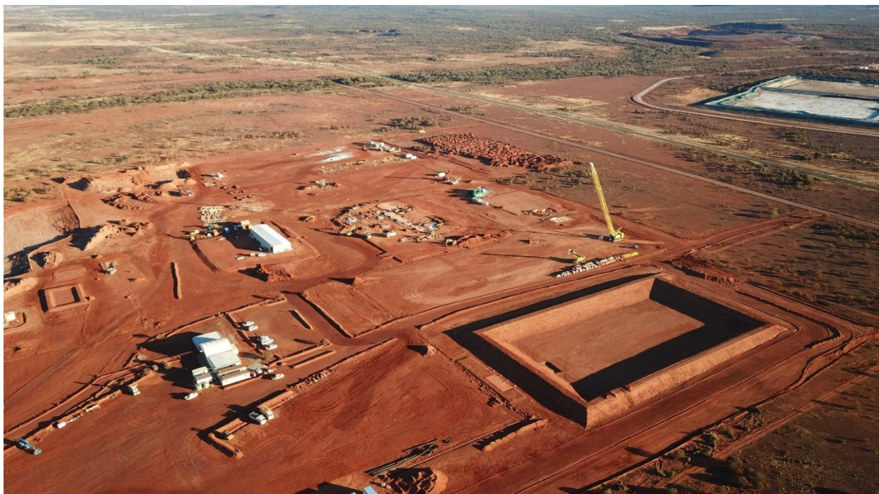
Figure 14: Process Plant / NPI construction site
