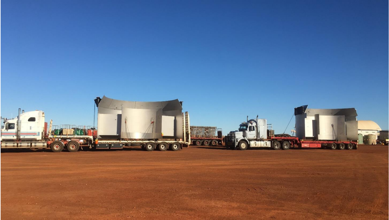
Figure 11: Crystalliser components at site
