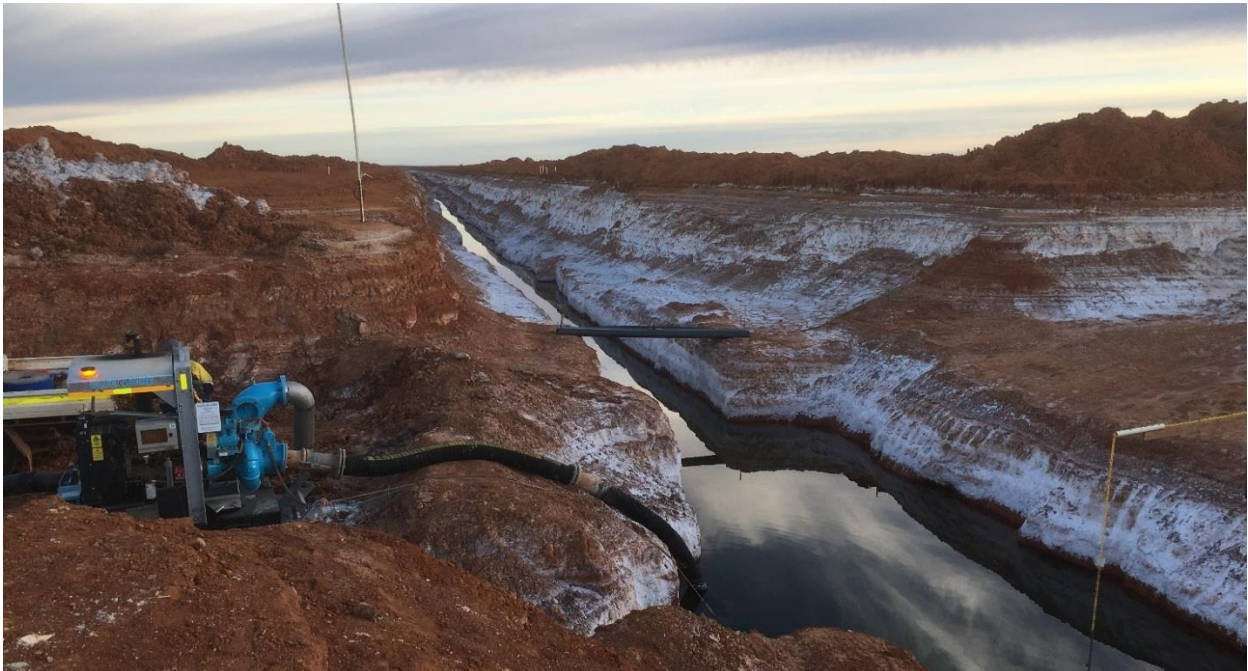
Figure 1: Trench Network Sump 1
