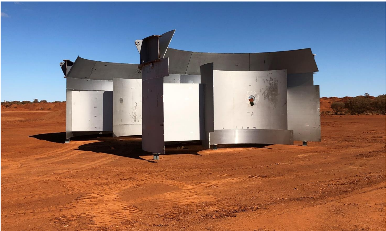
Figure 12: Crystalliser components at site
