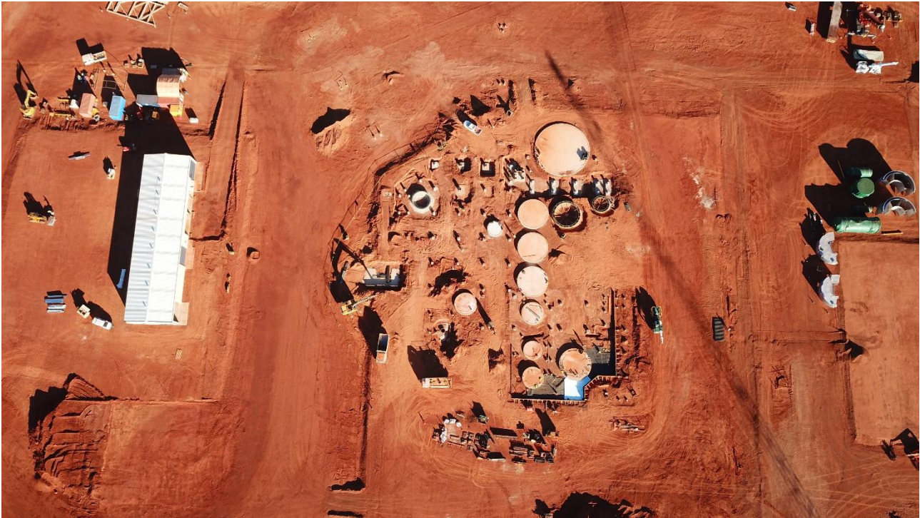
Figure 9: Process Plant concrete foundations
