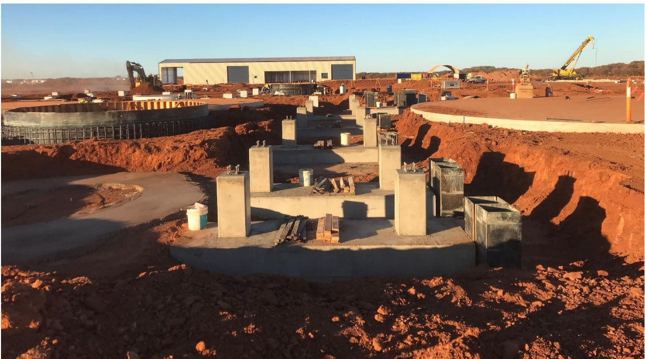
Figure 10: Process Plant concrete foundations
