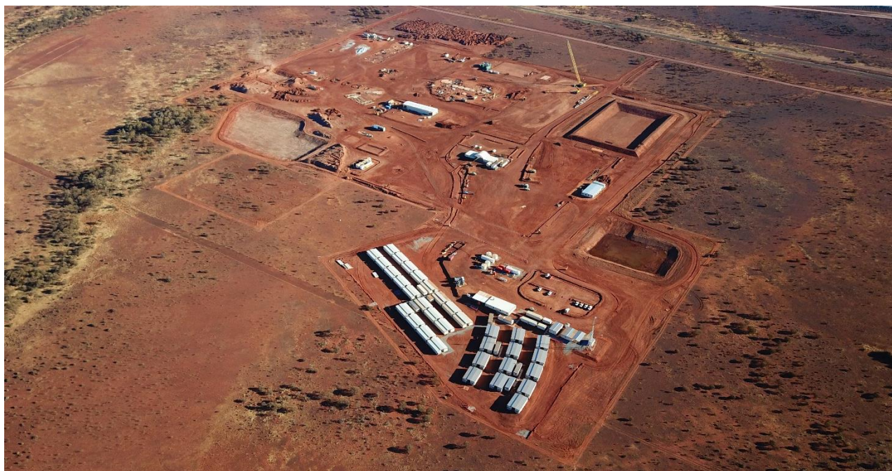
Figure 8: Process Plant construction site and Lake Way village
