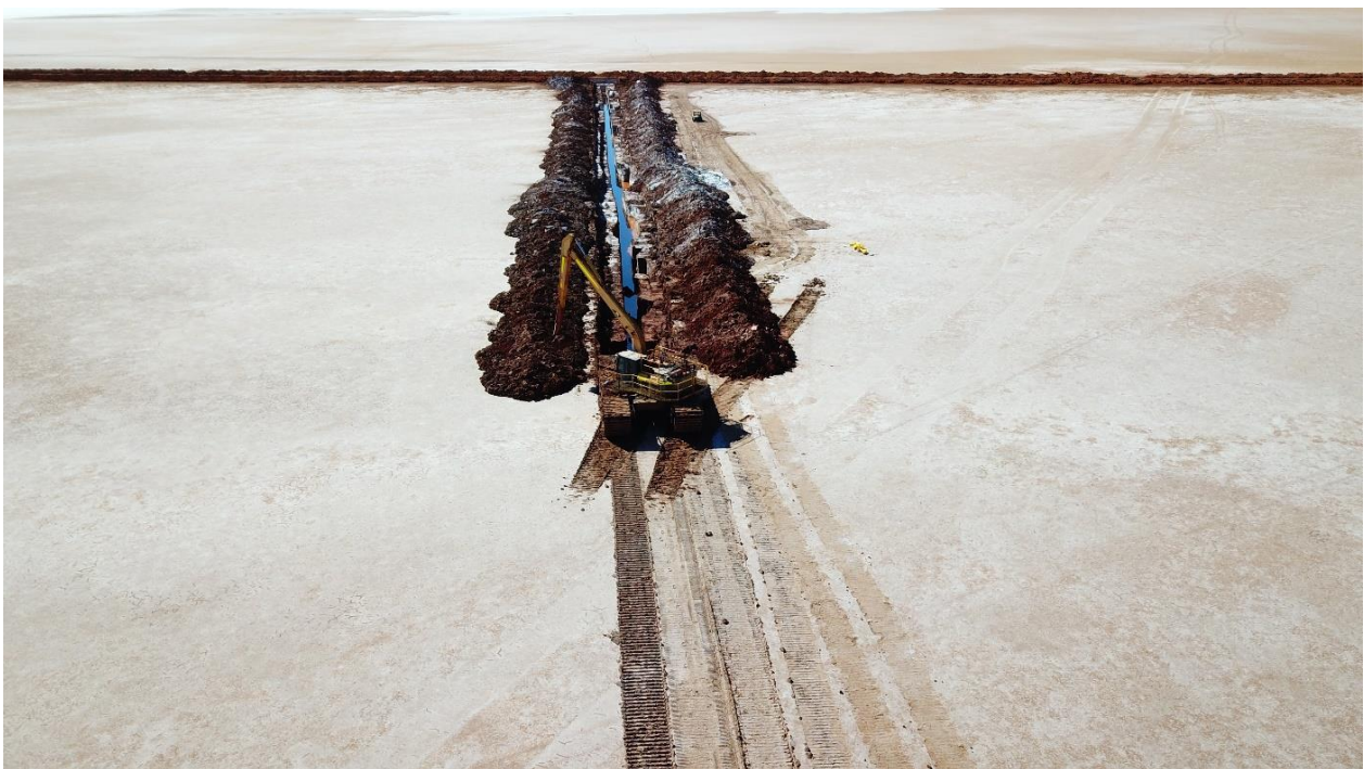
Figure 2: Trenching re-commenced during the quarter
