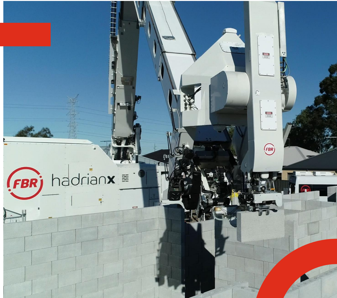
Hadrian X® completes its first house build in a residential development.
