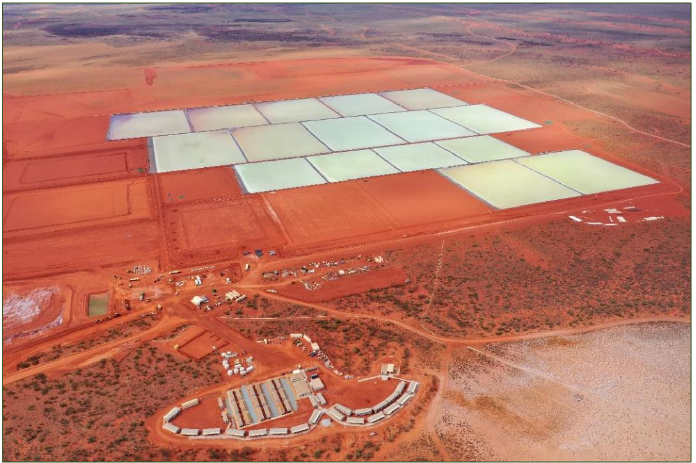
BSOPP Accommodation Village and Crystalliser Ponds - June 2020
