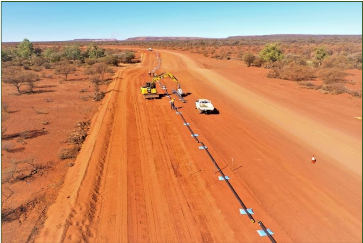
Gas pipe being placed along the access road to the Beyondie SOP Project
