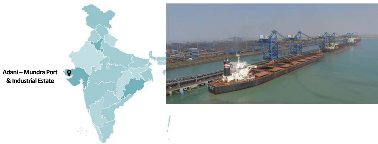
Figure 8 – Proposed Project Location adjacent to Mundra Port, the largest port in India
