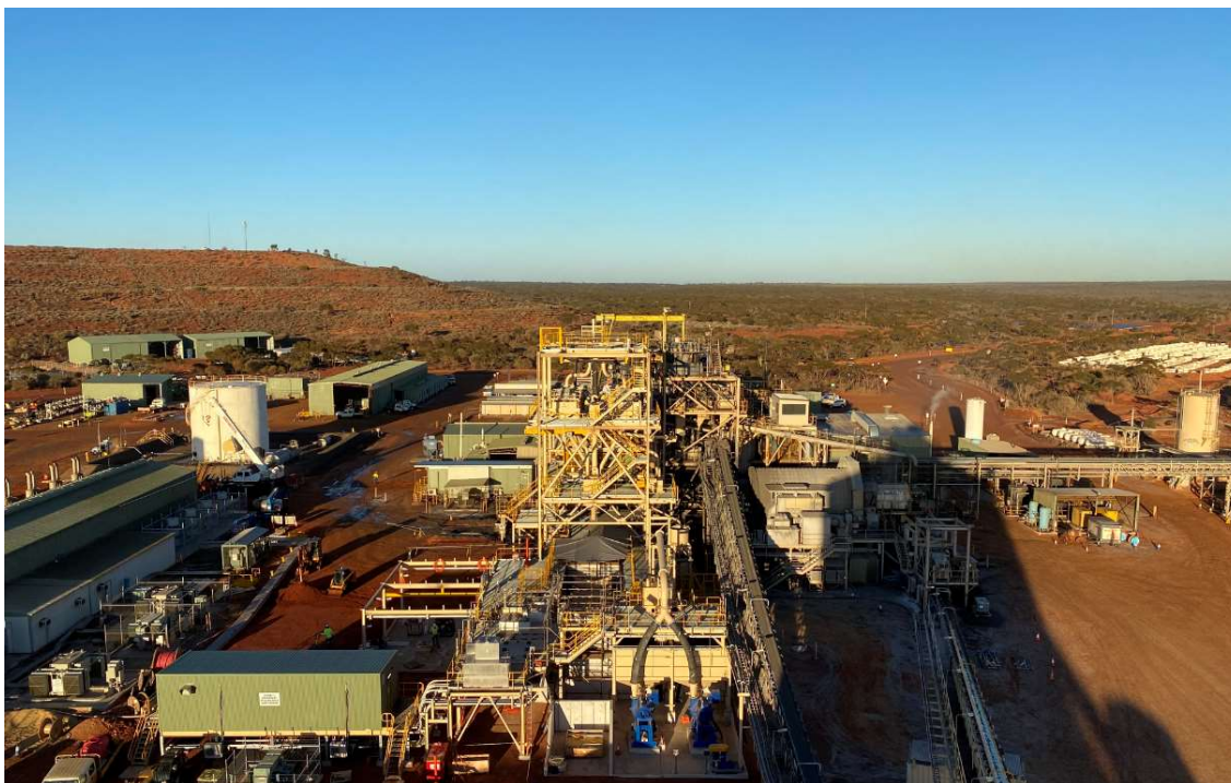
Figure 14 - Carosue Dam mill expansion continues
