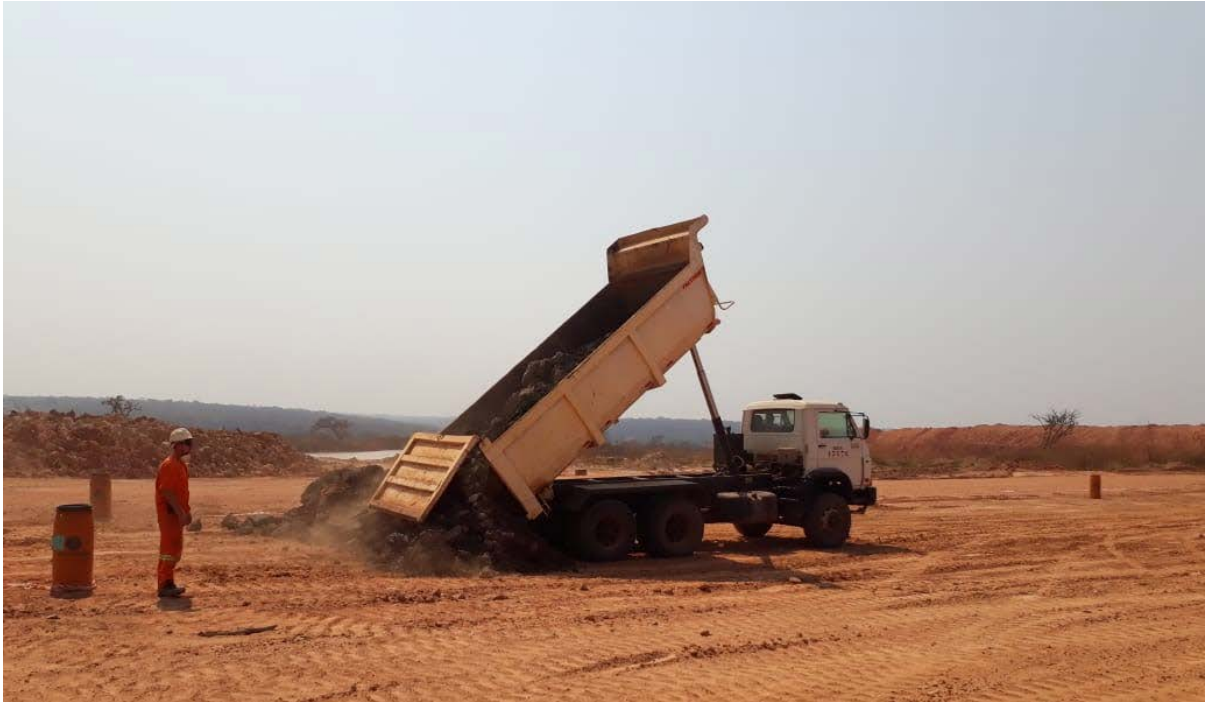
Delivery of the L071 kimberlite samples to the plant stockpile area
