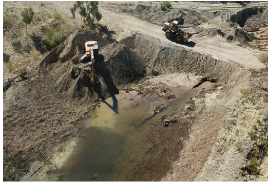
Figure 7. Construction of the Mt Freda Evaporation Pond.
