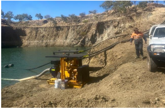
Figure 6. Field crew checking on pump station 1.
