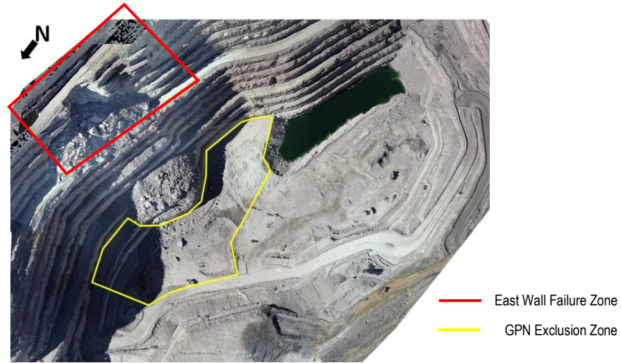
Figure 13 - Fimiston Pit, East wall failure zone and Golden Pike North safety exclusion zone
