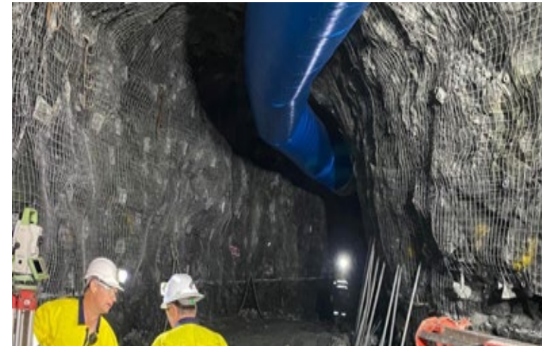
Underground development at Wiluna Mining Centre
