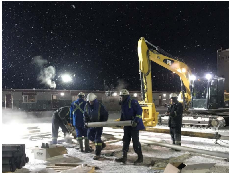
Figure 1 – Recovering core from the Calima-1 vertical well.
