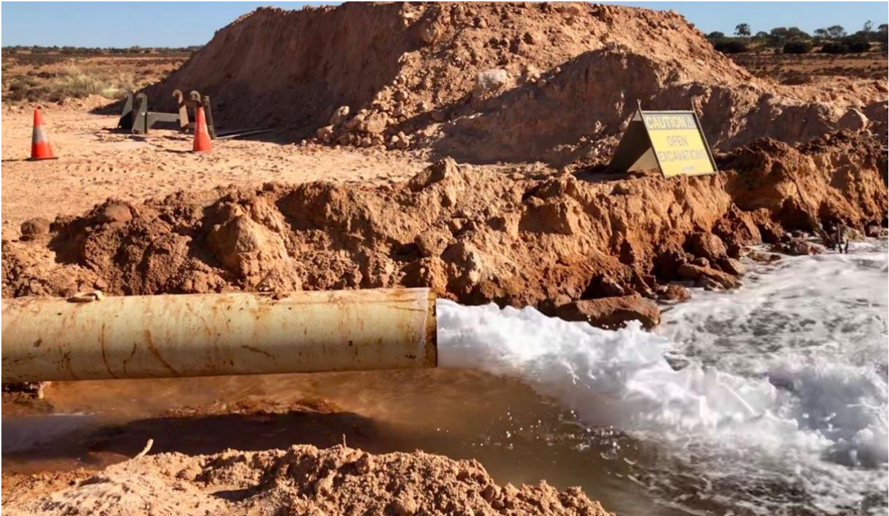
Figure 11: Airlifting at Pad 14
