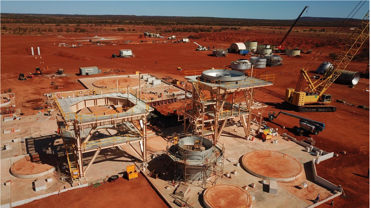
Figure 3: Schoenite crystalliser and SOP crystalliser structures
