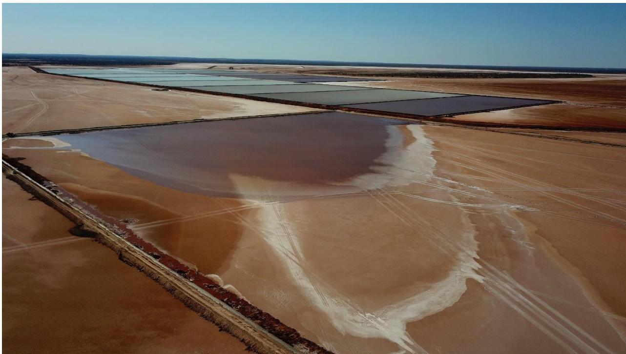
Figure 9: Construction of fourth pond train underway
