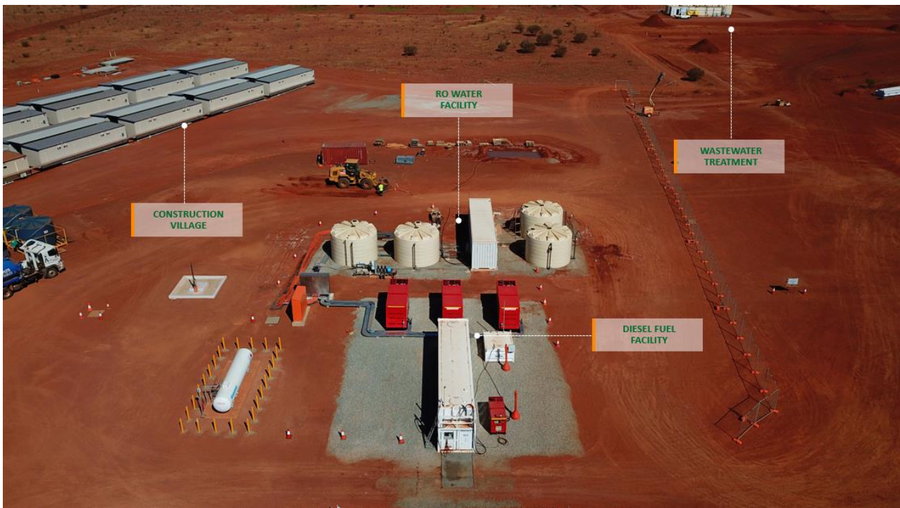
Figure 6: Diesel fuel and RO water facility
