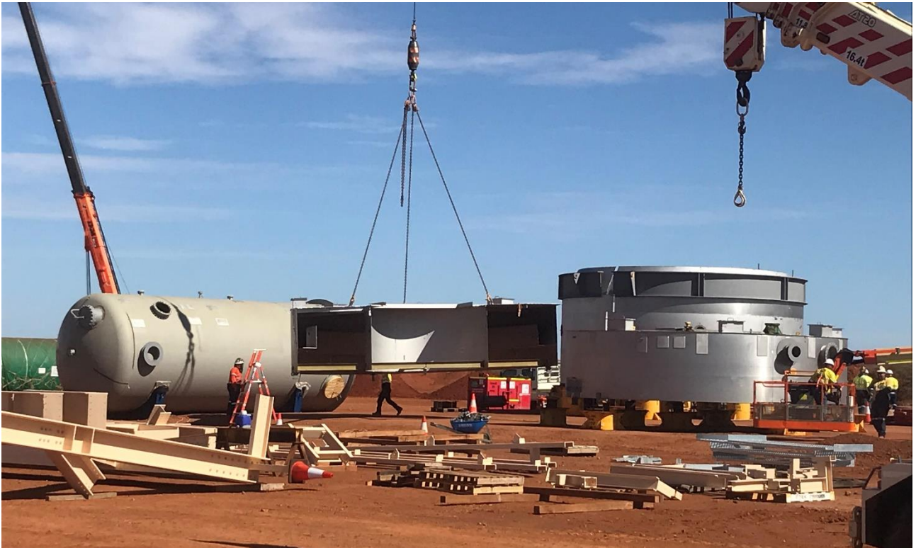
Figure 7: Process Plant crystalliser being installed on site
