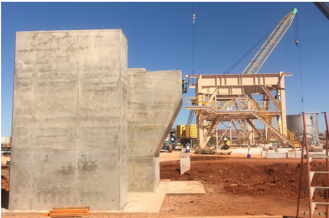
Figure 5: Rotary dryer foundation and crystalliser steelwork
