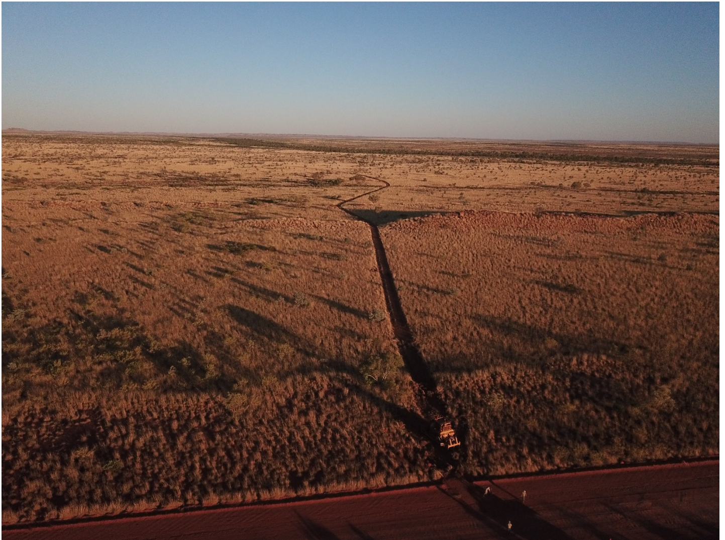
New access road construction commenced
