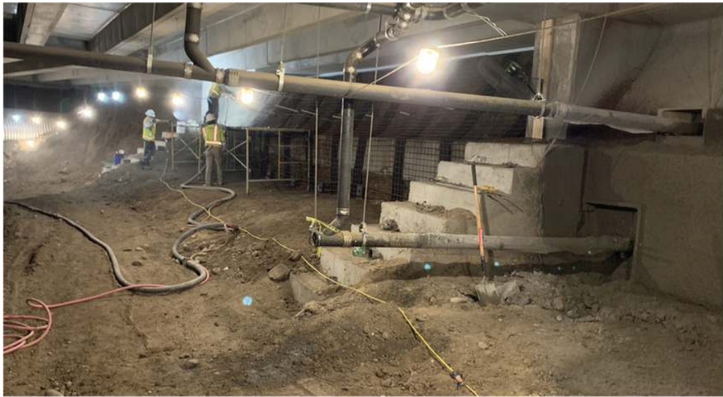
Figure 6. Shotcrete (including EdenCrete®) used in in Health, Nutrition and Physical Therapy Centre
