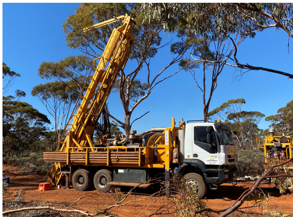
Figure 3 – 28 August 2020 RC Drilling on site
