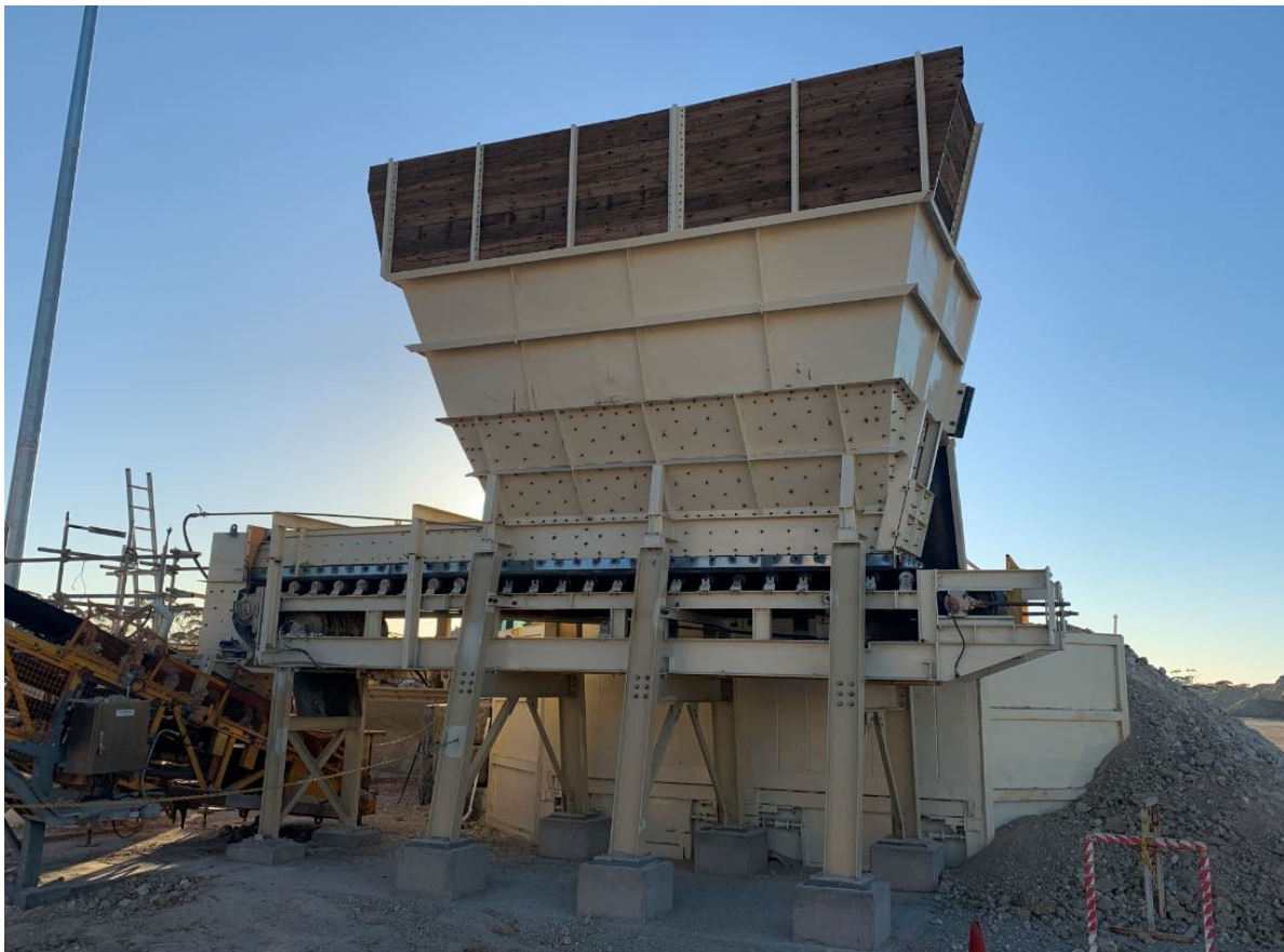
Figure 1: Jaurdi Gold Project - Feed Hopper and Belt Feeder
