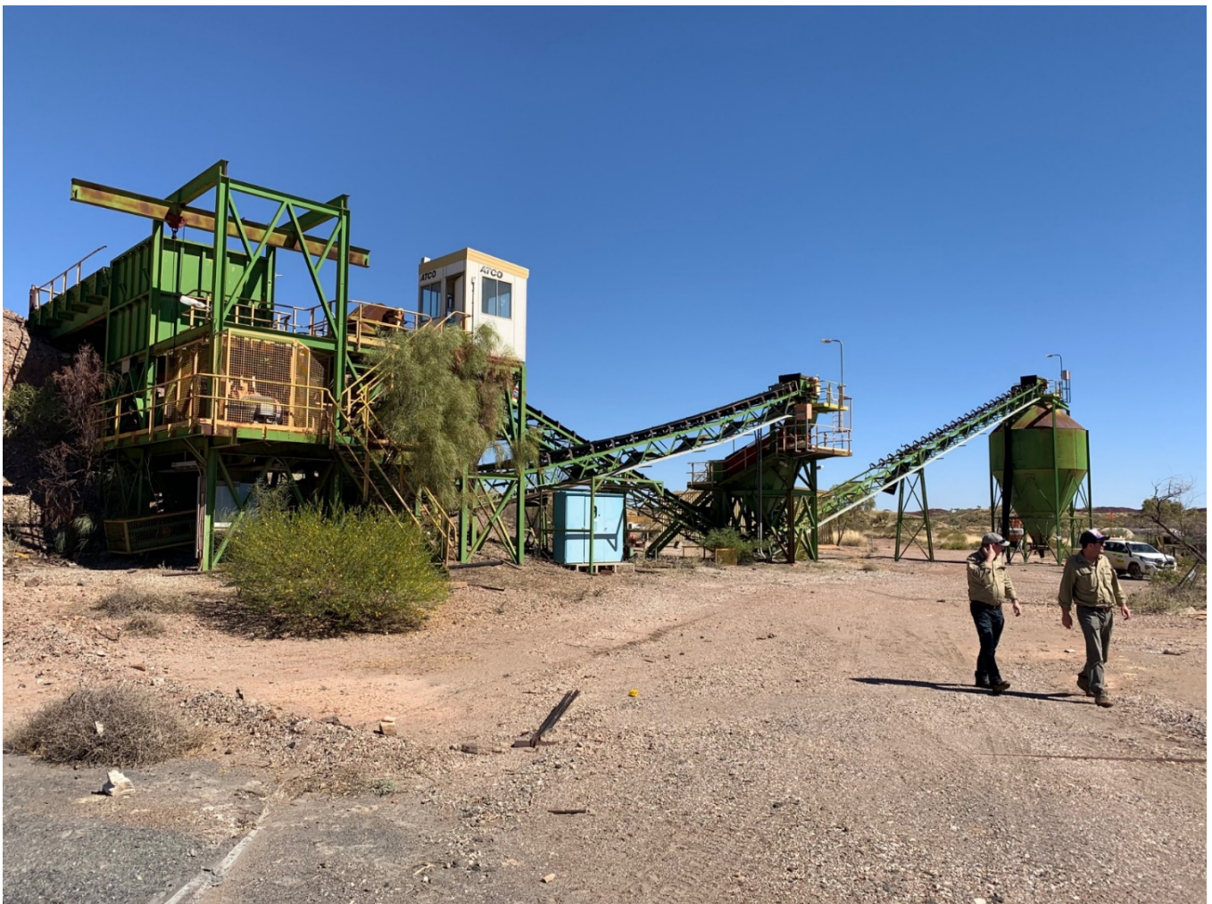
Figure 7: Existing crushing plant
