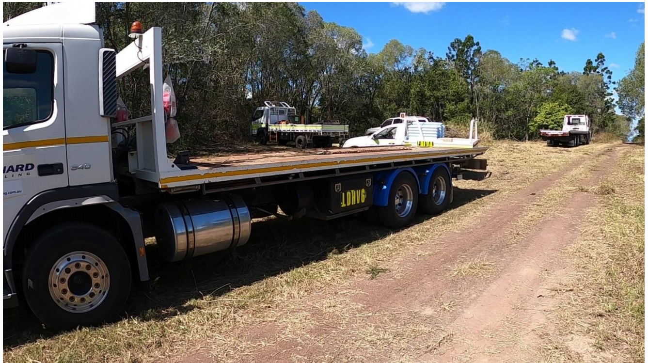
Mobilising equipment for the Stage 2 diamond drilling program
