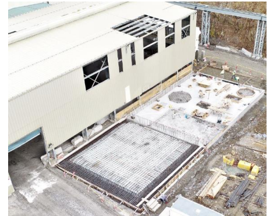
New Tailing Filter Civils
