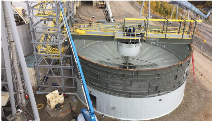
New Tailing Thickener construction
