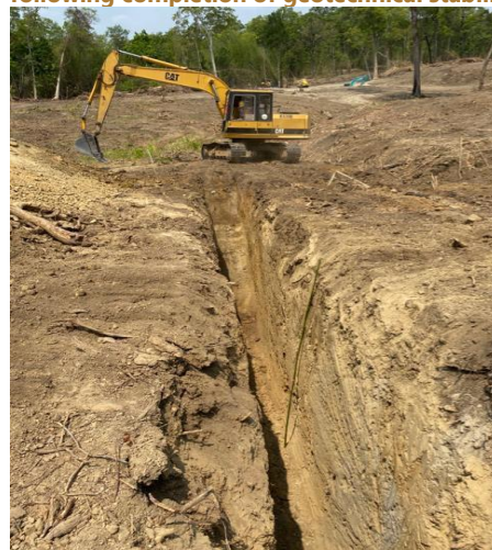
Figure Seventeen | Plant site cleared and topsoil pushed up following completion of geotechnical stability assessment
