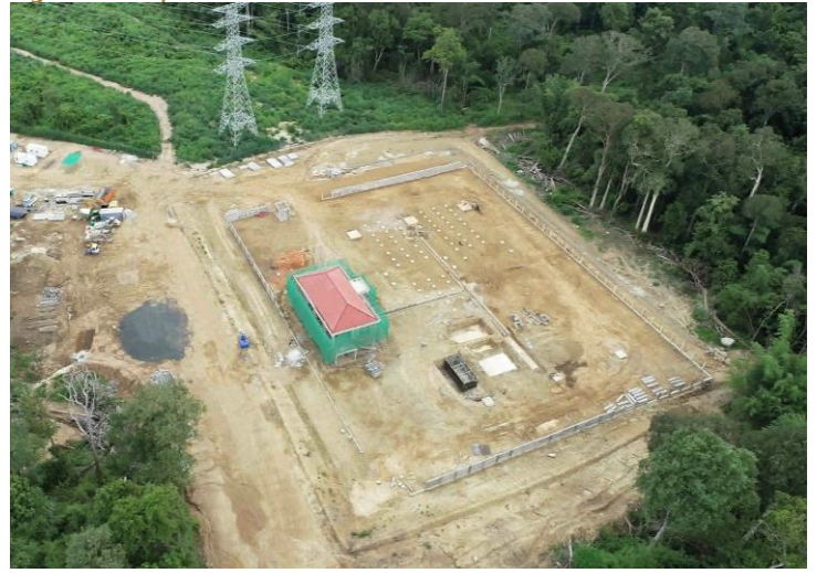
Figure Seven | Substation Civil Works Aerial view
