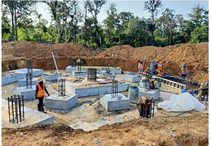
Figure Thirteen | Float Cell Foundation
