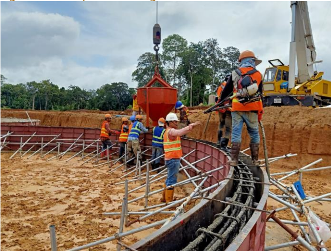
Figure Fourteen | CIL Tank Ring beams
