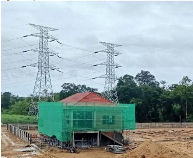
Figure Six | Substation Civil Works
