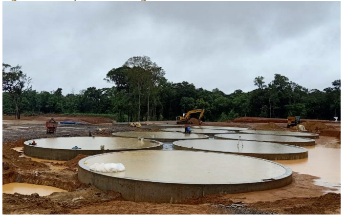
Figure Fifteen | CIL Tank Ring beams
