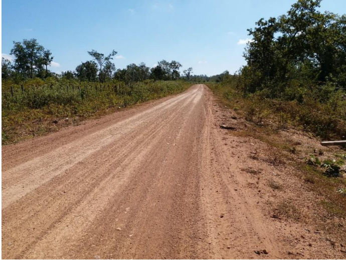
Figure Four | Okvau Access Road
