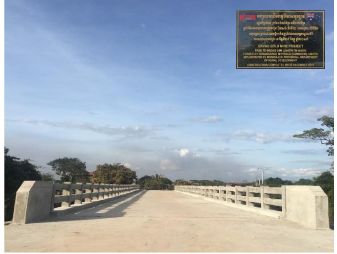
Figure Five | Prek Te River Bridge
