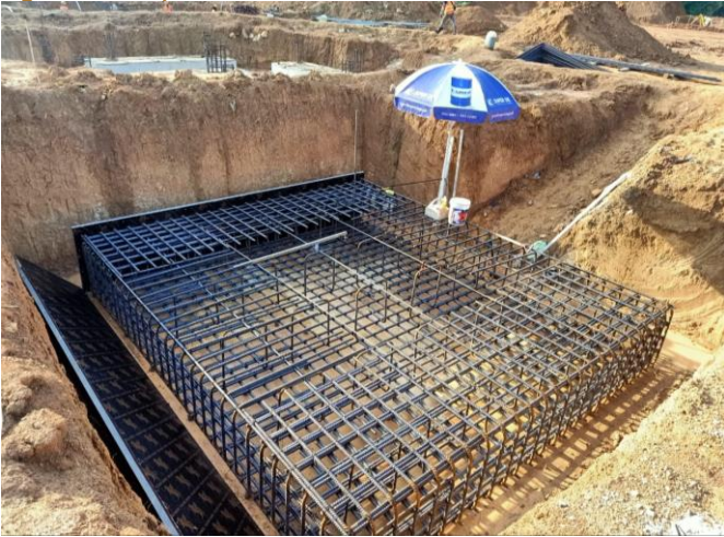
Figure Twelve | HIG Mill Foundation
