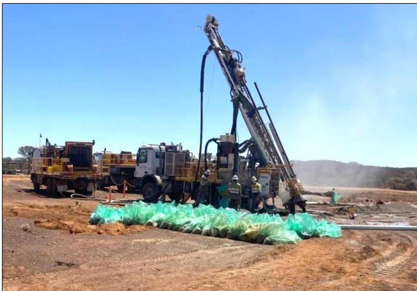
Figure 3. Strike Drilling truck-mounted RC rig drilling at the Melville Gold Project targeting down-dip and along-strike continuity of newly discovered mineralised position east of the main historic resource.
