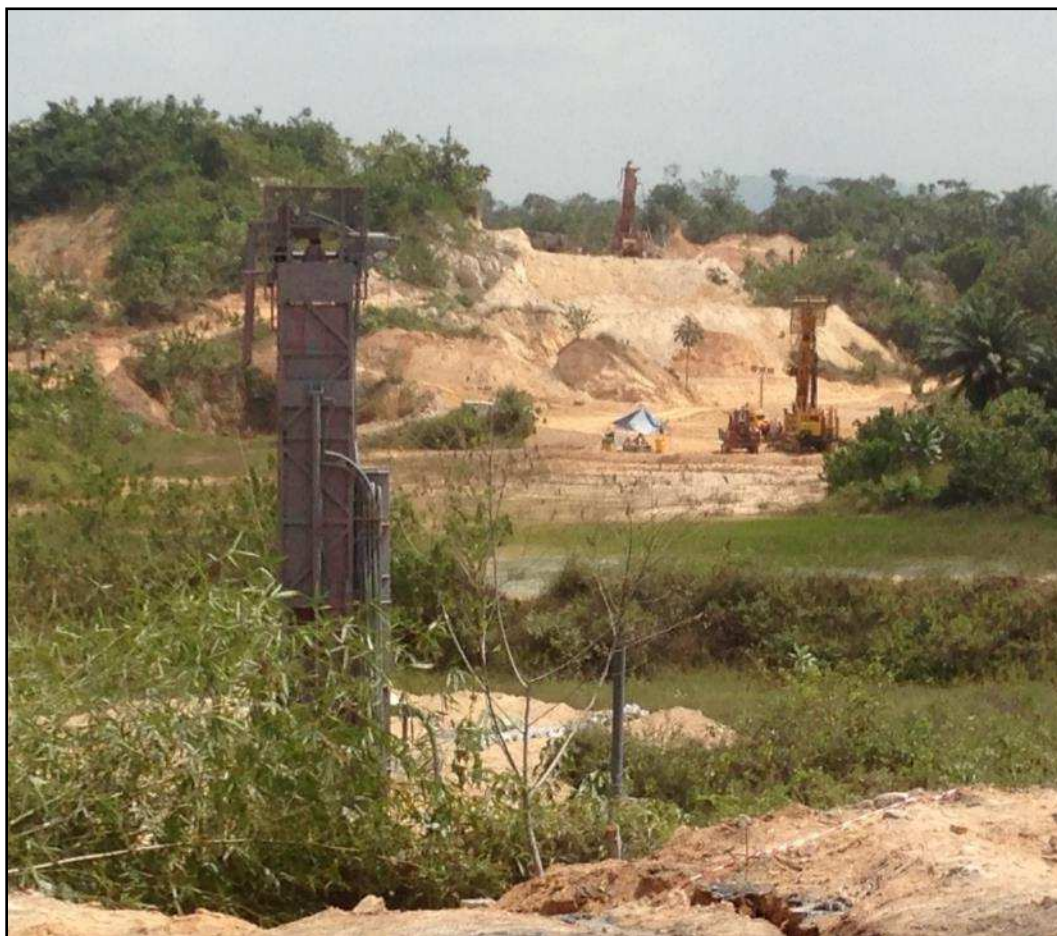
Drilling operations at Adiembra, February 2020
