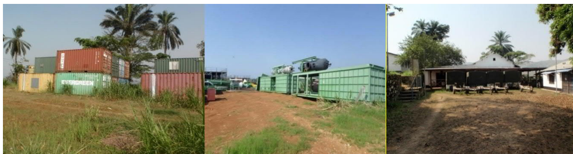
Figure 3, 4 and 5: Mechanical plant, equipment and storage and camp facilities at the Adidi-Kanga site
