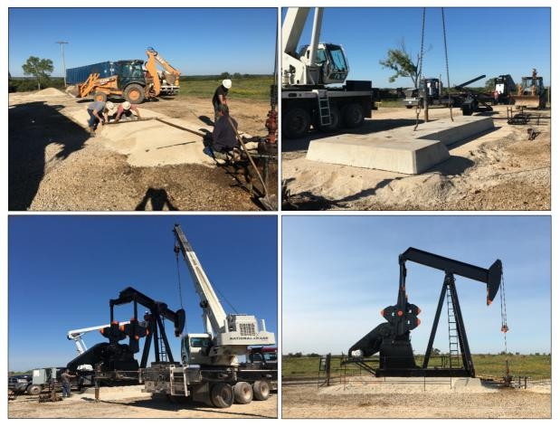
Pumping Unit being installed on the Mitchell 1-12 well, Carter County
