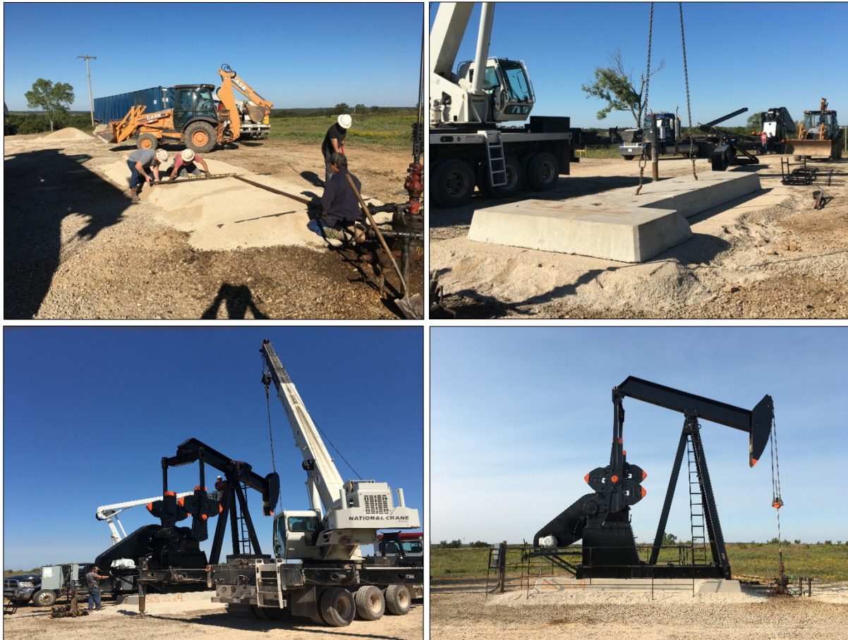
Pumping Unit being installed on the Mitchell 1-12 well, Carter County
