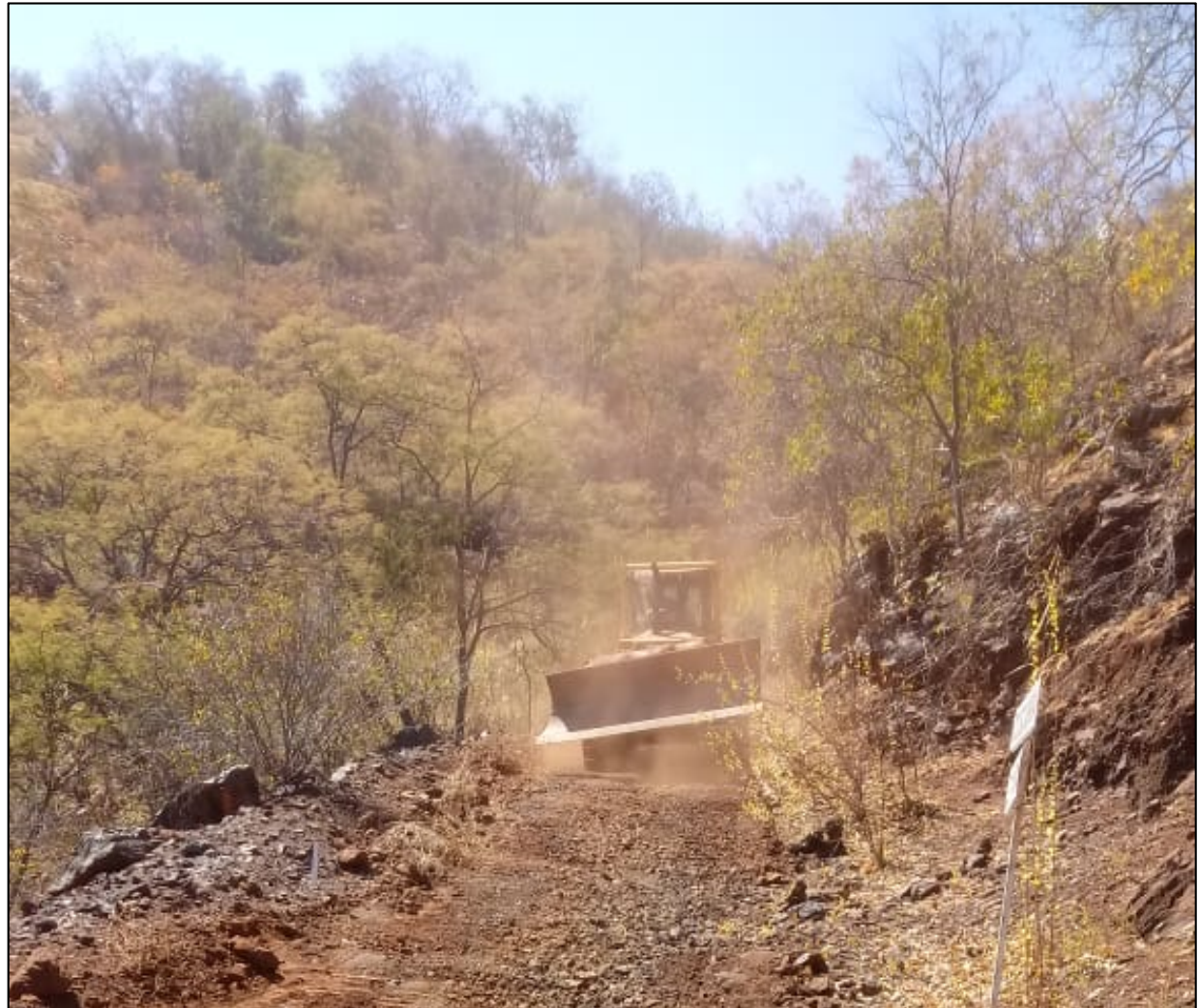
Drilling Road Preparation
