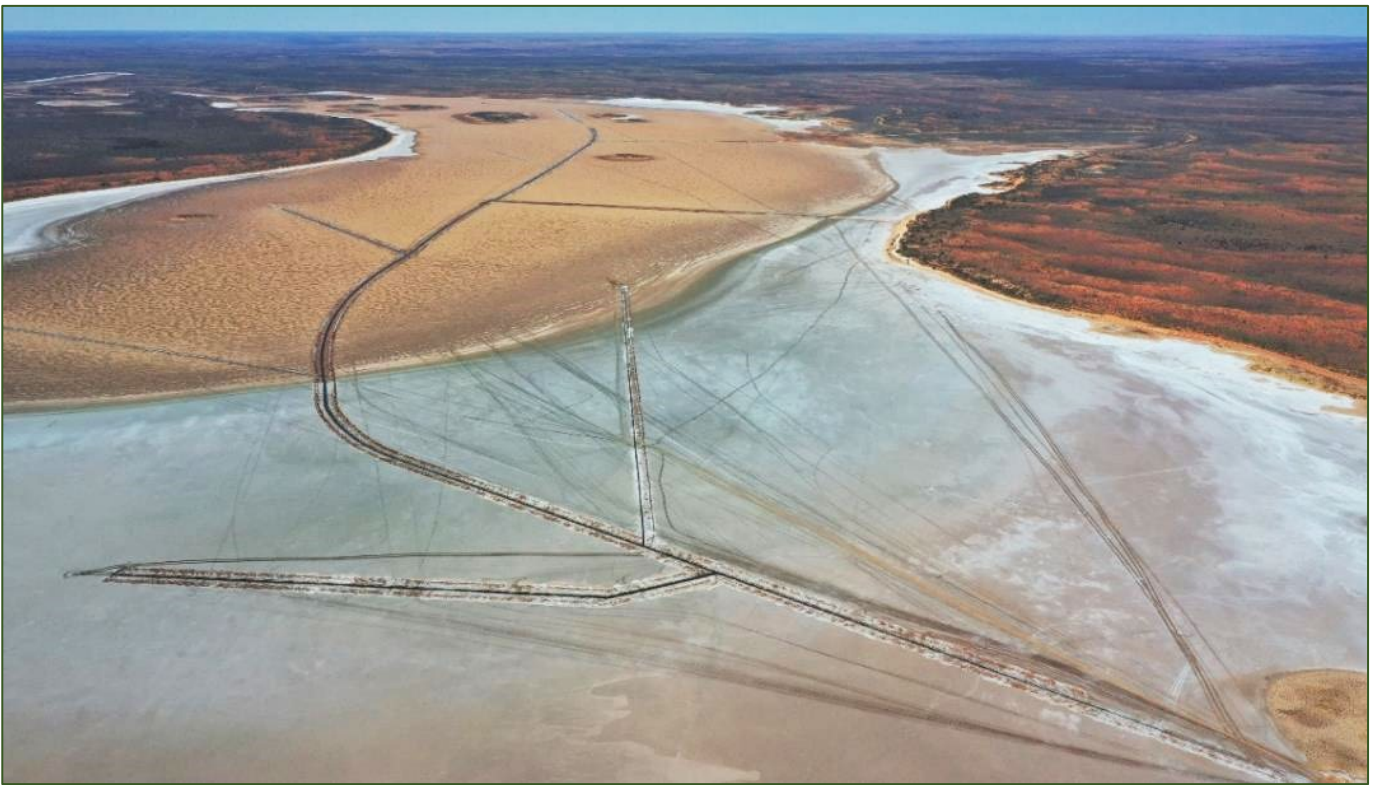
15 kilometres of trenches complete at Lake Sunshine
