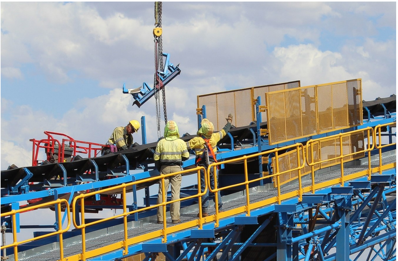
Figure 7: Rocklands Process Plant - major components installed, structural completion underway.
