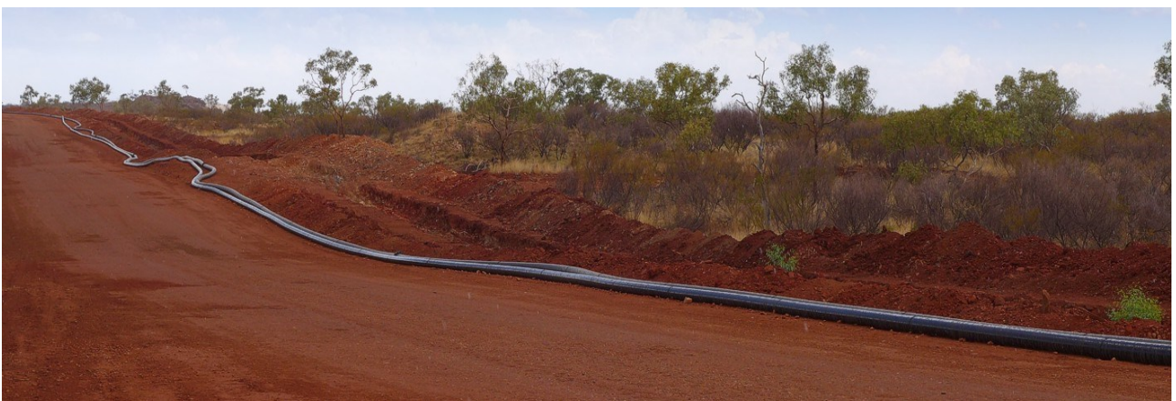
Figure 15: Mining commences at RS1 pit (top image); Equipment on the go-line at the TSF (middle image); and water pipes connecting the Tailings Storage Facility (TSF) to the Process Plant ready to be installed in trenches (bottom image).,
